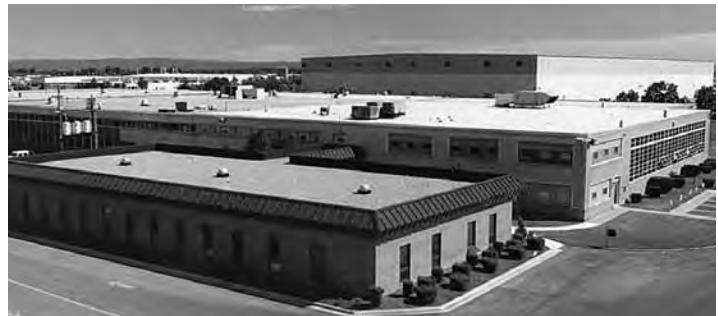
Ashworth's Manufacturing Facility—Winchester, Va.
